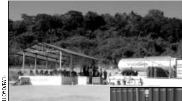
The VidaGas plant on its launch day and (inset) a burner and lamp for domestic use
